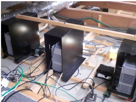
(c) Installation of cameras and projectors on the ceiling
